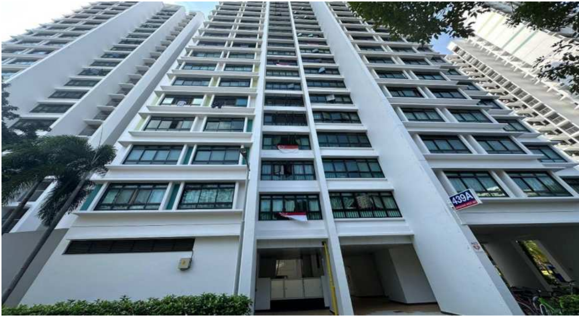
Newly painted residential blocks at Blks 430A – 430D, 436A – 436D, 438A – 439C, 440A – 440C Fernvale Road
