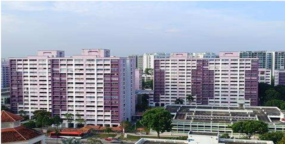
Newly painted residential blocks at Blk 552 to Blk 566 Hougang St 51
