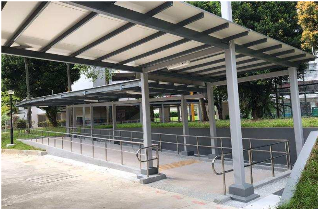
Sheltered barrier free access linkway at Blk 180 Ang Mo Kio Ave 4
