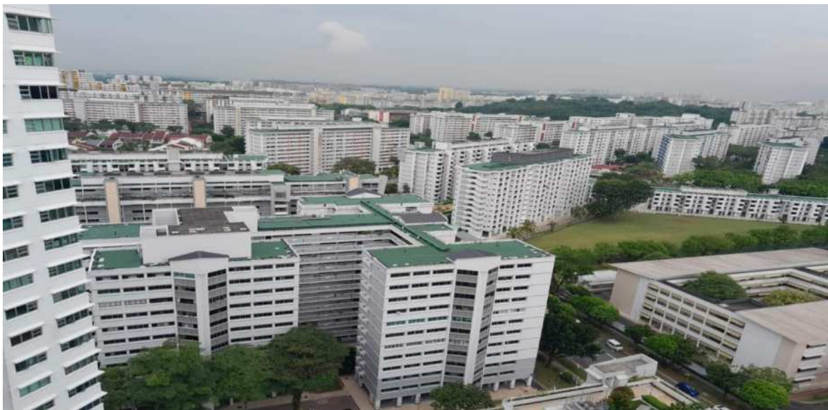
Re-roofing works at Blk 158 Ang Mo Kio Ave 4
