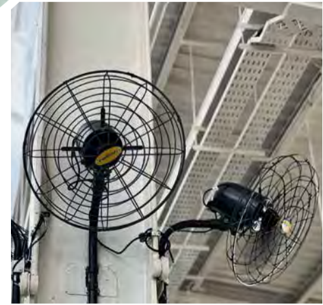
SOME OF THE UPGRADES: (From top) Improved accessibility for wheelchair users, upgraded tables and chairs, refurbished restrooms, better ventilation and new wall fans.
