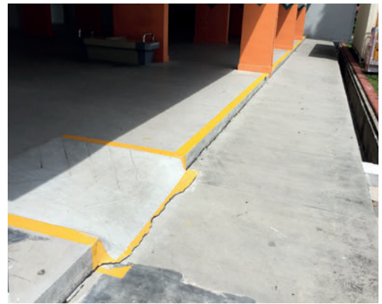
Yellow strips along the pathway to alert residents to the kerb.
