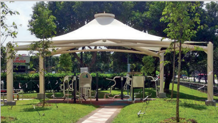
Tensile membrane shelter at existing fitness corner at Block 615 Hougang Avenue 8
