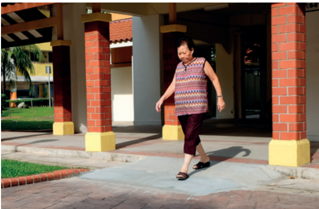
Ramps installed where there is a difference in levels for better mobility.
