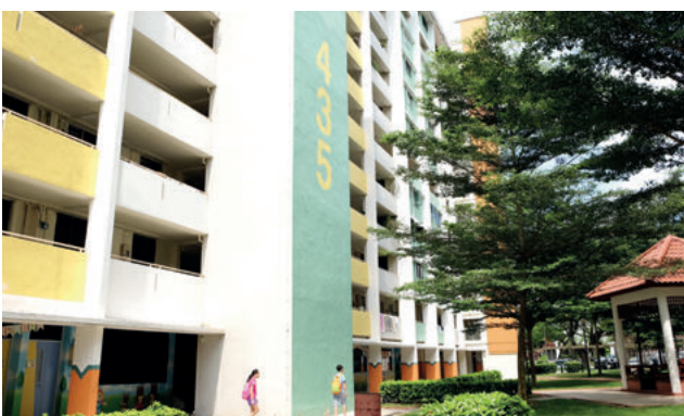
Block numbers are painted large on the buildings and ensured that they are not blocked from view.
