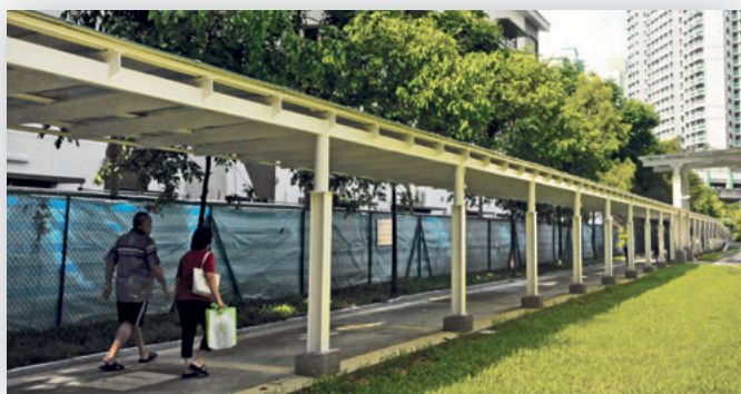
Low covered linkways from the Barrier Free Accessibility ramp next to Block 441D to Block 441C and 445A Fernvale Road
