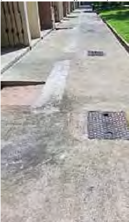
Here is the foot of Block 647, freshly cleaned (for the second time in a day) at about 3pm...
